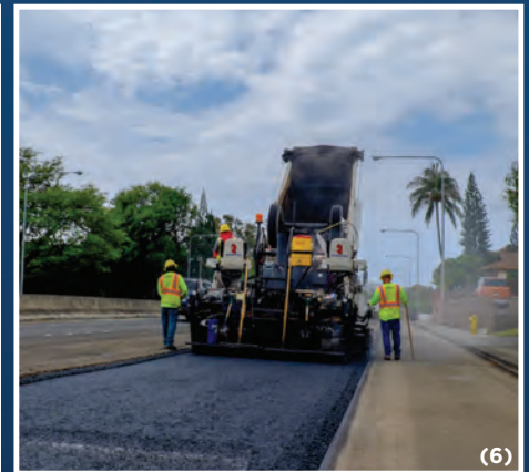
(4) Grade "A" Aggregate at Makakilo Quarry (5) Truck loads paver with Hot Mix Asphalt (6) Paving Kalaniana'ole Highway
