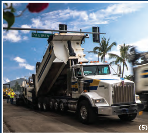
(4) Grade "A" Aggregate at Makakilo Quarry (5) Truck loads paver with Hot Mix Asphalt (6) Paving Kalaniana'ole Highway
