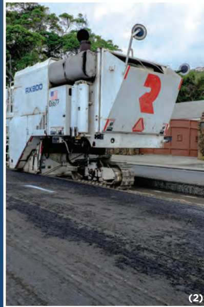
February 2015 repaving of Kalaniana'ole Hwy., Niu Valley. Existing material is removed (cold-planed) and repurposed before repaving. (1) and (2) Cold-planer removing top surface of existing roadway (3) Resulting material loaded into trailer for transport.
