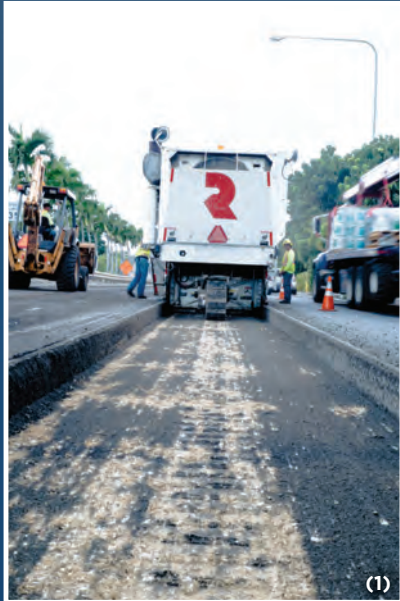
February 2015 repaving of Kalaniana'ole Hwy., Niu Valley. Existing material is removed (cold-planed) and repurposed before repaving. (1) and (2) Cold-planer removing top surface of existing roadway (3) Resulting material loaded into trailer for transport.
