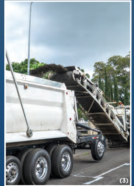
February 2015 repaving of Kalaniana'ole Hwy., Niu Valley. Existing material is removed (cold-planed) and repurposed before repaving. (1) and (2) Cold-planer removing top surface of existing roadway (3) Resulting material loaded into trailer for transport.
